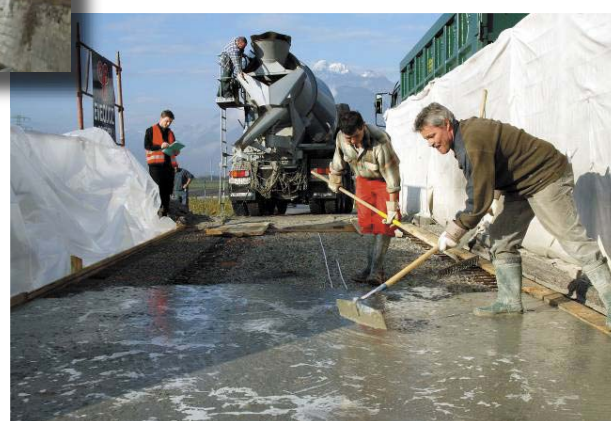
This full scale realization in realistic site conditions clearly demonstrates that the technology of UHPRFC is now mature for cast in-situ applications of rehabilitation, using standard equipments.
