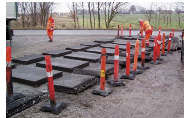
Samples of pavement to be tested in the laboratory.
