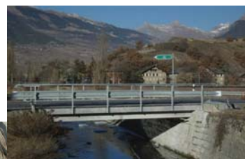
This full scale realization in realistic site conditions clearly demonstrates that the technology of UHPRFC is now mature for cast in-situ applications of rehabilitation, using standard equipments.
