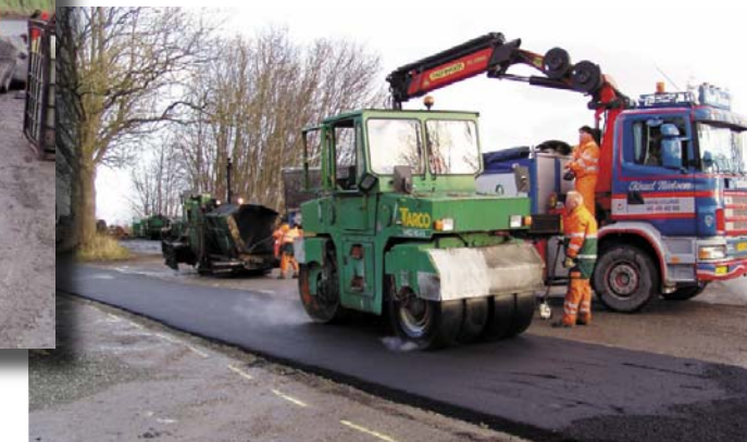
Construction of pavement consulting of alternative materials.
